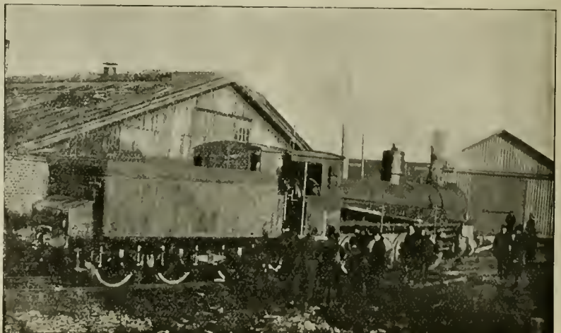
READY FOR THE TEST.
